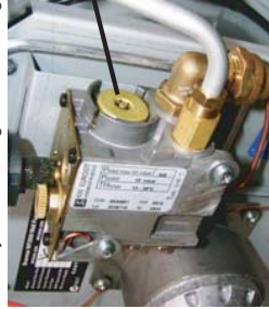
CLOCKWISE: Increase pressure ANTI-CLOCKWISE: Decrease pressure
