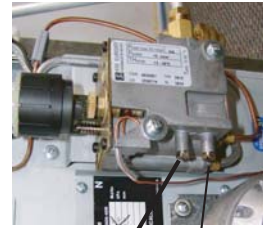
BURNER PRESSURE TEST POINT (Use 8mm spanner or blade screwdriver)
